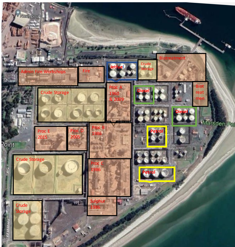
Figure 25: Marsden Point storage
