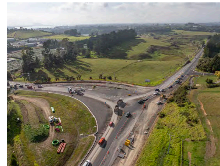
SH2 Ōmokoroa interchange site
