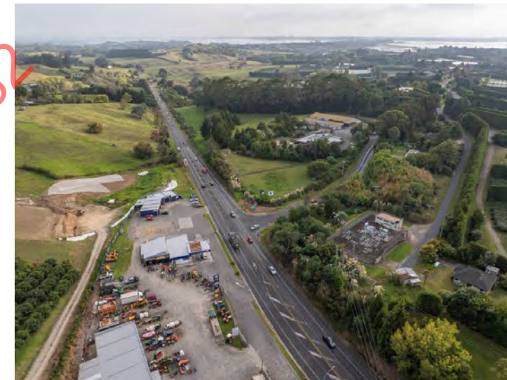
Substation site, Plummers Point Road
